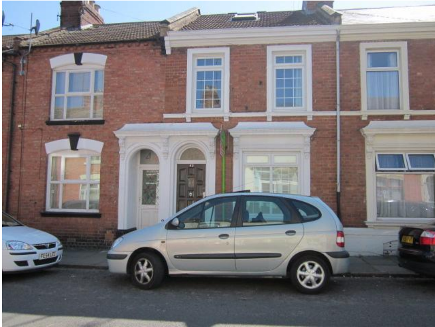
General view of the property
